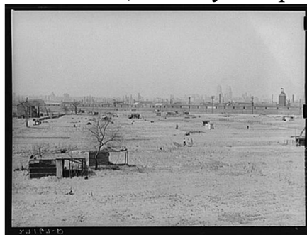
Squatters' houses in "Jersey Meadows," on city dump
